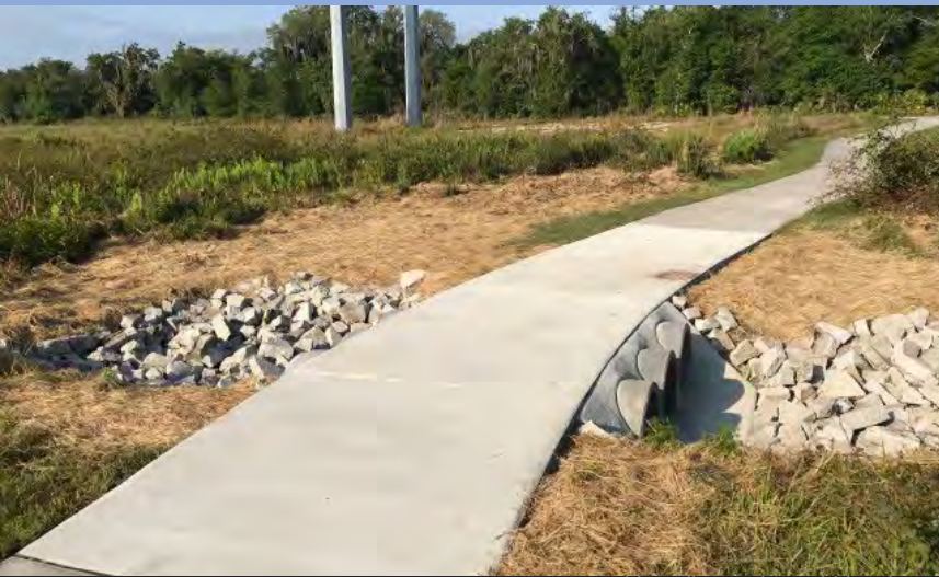
Sidewalk Repairs at Fishhawk Ranch CDD
