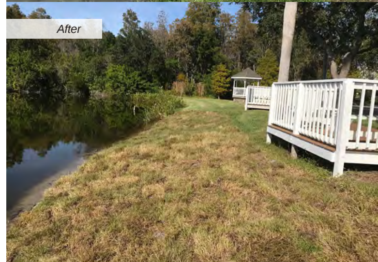
Pond Restoration at Westchase CDD
