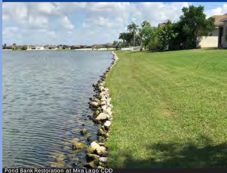
Pond Bank Restoration at Mira Lago CDD
